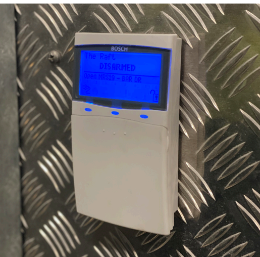
Multiple Bosch Solution 6000 proximity keypads & Professional Series detectors were installed around the venue.
