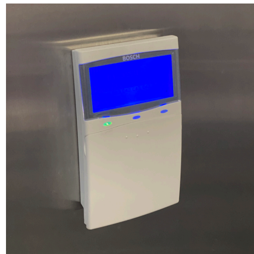
Multiple Bosch Solution 6000 proximity keypads & Professional Series detectors were installed around the venue.
