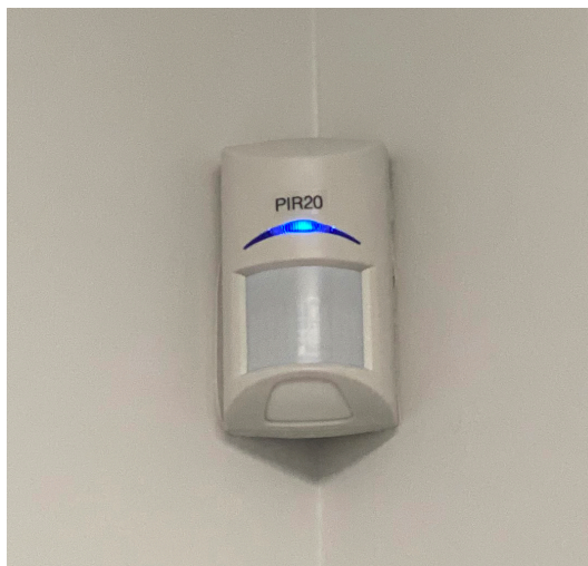
Multiple Bosch Solution 6000 proximity keypads & Professional Series detectors were installed around the venue.
